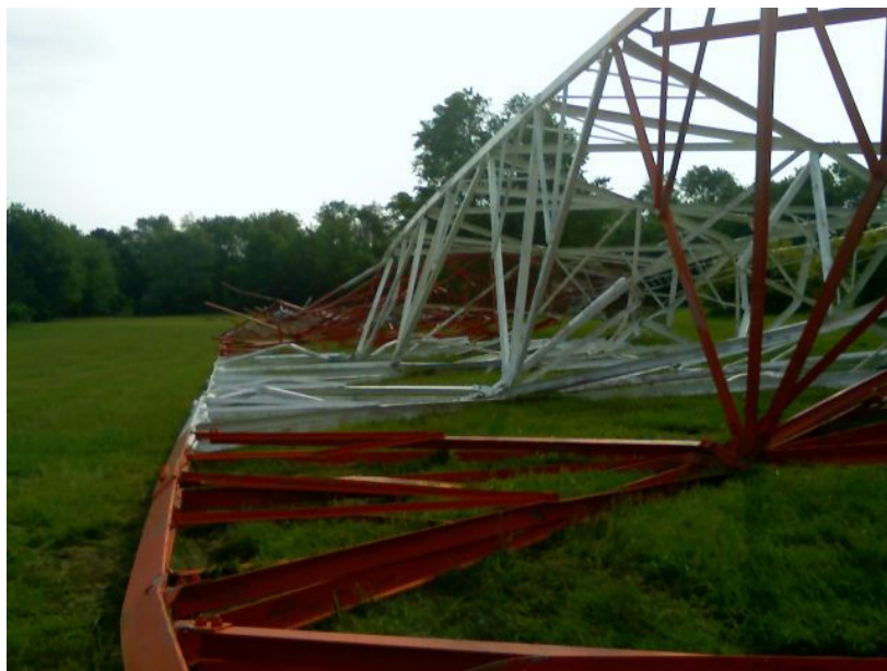
Remember the Ch 17 tower in Louisville? This is what was left after they torched it. Luckily, they were able to drop it with no harm to people, or Property. TNX to K80MO for the picture
