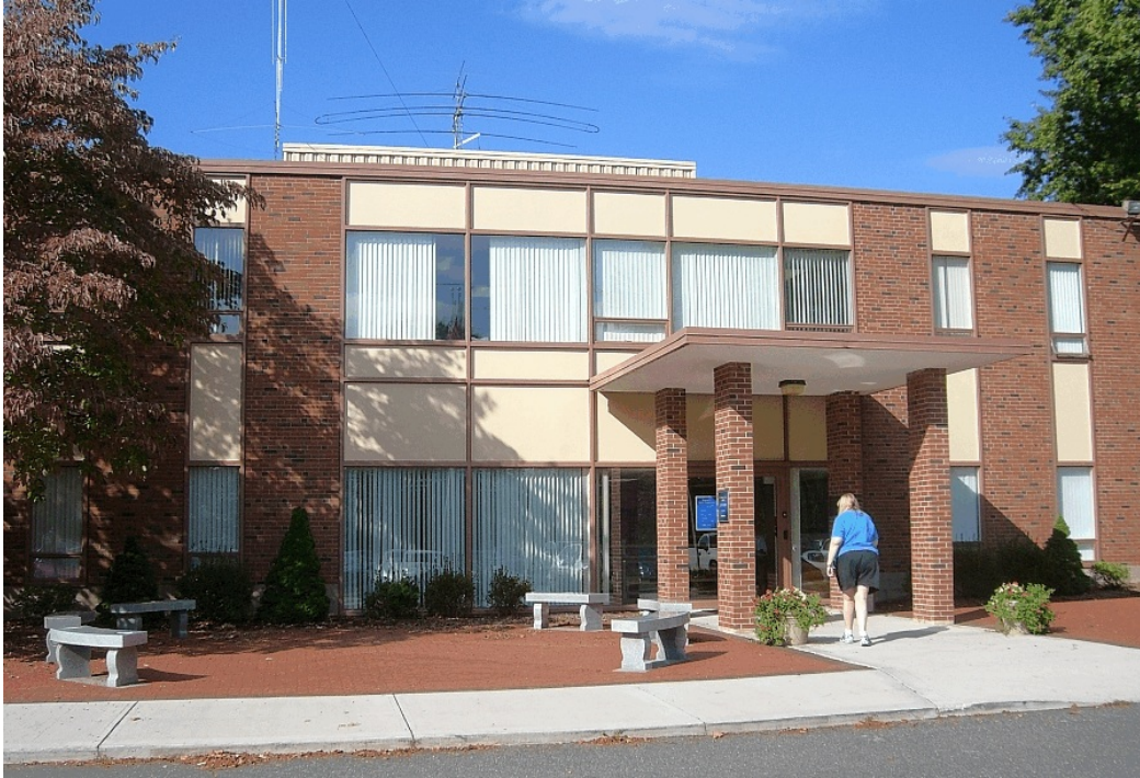
ARRL HQ front entrance
