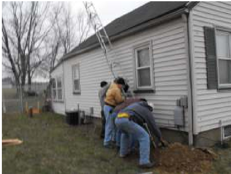
Here's the tower sliding ever so gently into the hole.
