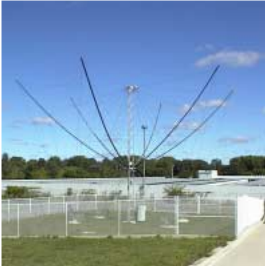
This is the Multi band antenna at FEMA Headquarters in Columbus. I think they said the bandwidth was "DC to daylight," or something like that.
